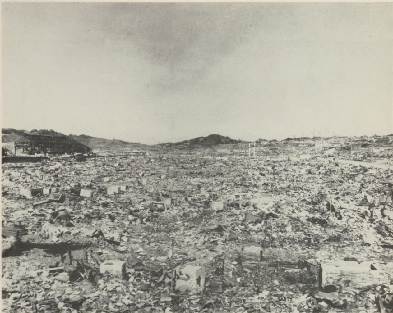
Photo 1. 2500 feet south of GZ. Looking north. Total damage by blast and fire.
